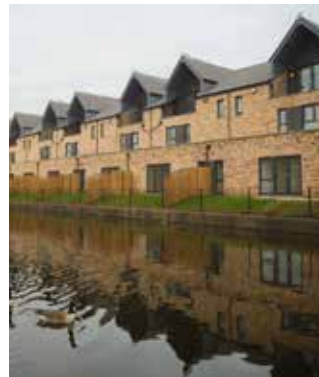
The Dob Brook Close scheme in Newton Heath, completed by Guinness Partnership in October 2022
